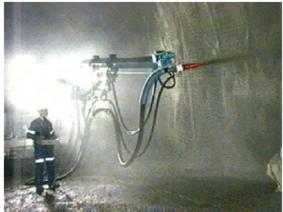
Fig 9. Robojet in operation
