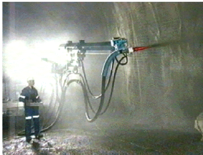
Fig. 13 - Robojet in operation
