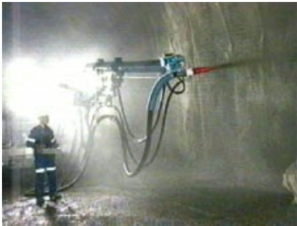
Fig.6: Robojet in operation
